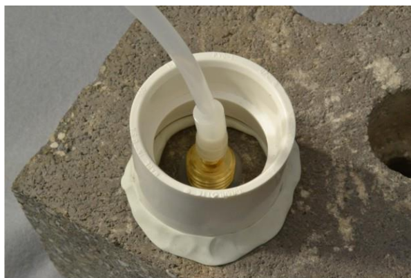
Figure 8. Water dam used for leak detection
