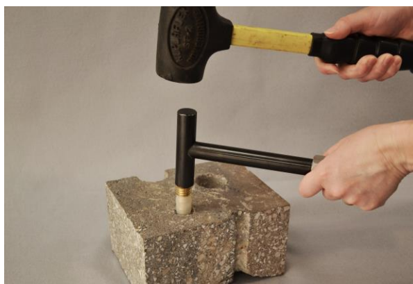
Figure 2. Installing the Vapor Pin™.
