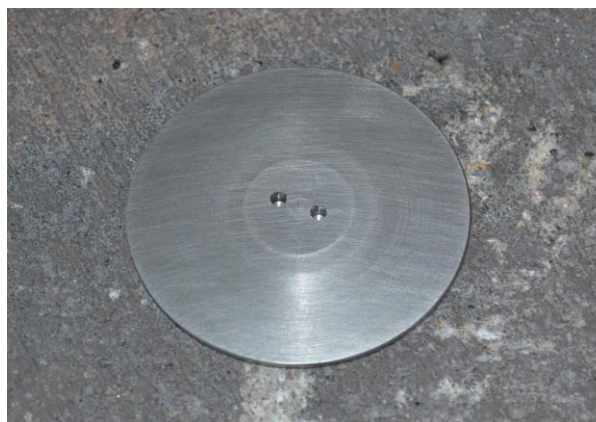
Figure 4. Secure Cover Installed
