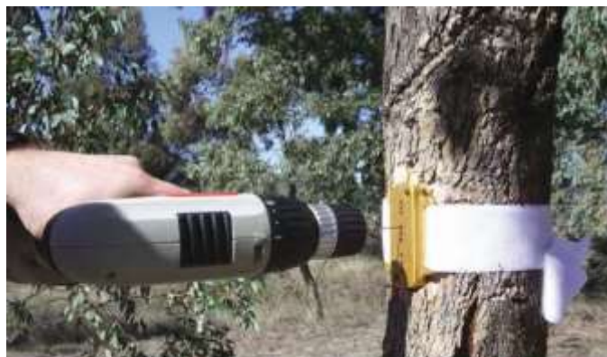
Photo 29: Horizontal drilling using a conventional cordless drill.
