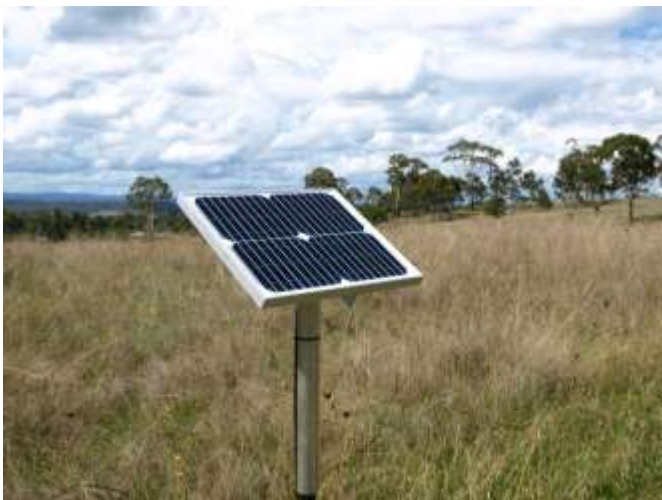
Photo 5: SP22 Solar Panel mounted to star picket.
