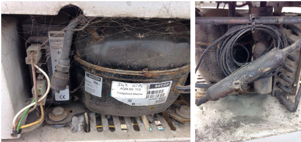
Figure 0-30 Dirt and debris can accumulate within the TMS cassette leading to reduced efficiency of the thermal management system.
