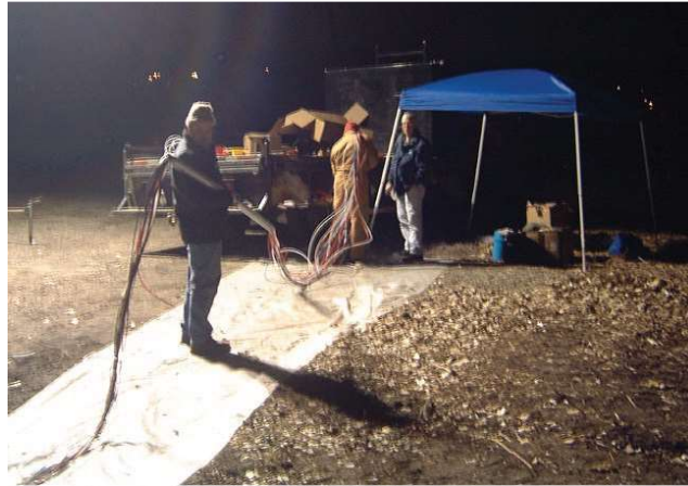
Figure 4-5 Casing Section Being Threaded Over Monitoring Tubing
