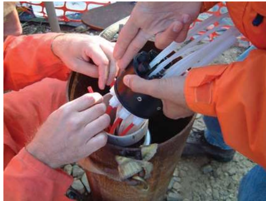
Figure 9-3 Pump Tubing Being Attached to a Wellhead
