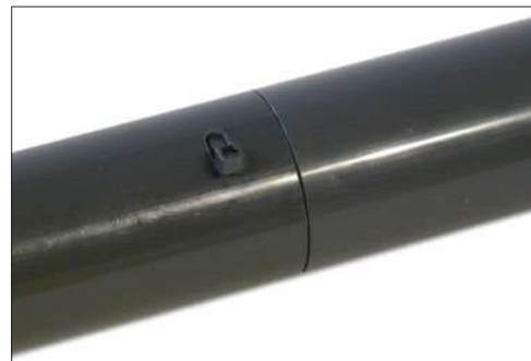
Figure 5-6 Cut Off the Excess Shear Tie
