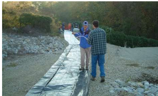
Figure 6-2 Tubing Being Pulled to Reference Mark
