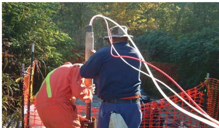
Figure 4-4 Initial Section Being Installed Down-hole
