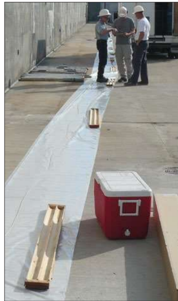
Figure 4-1 Plastic & SS Support Cable Laid Out (Wood core boxes are used here to weigh down plastic)
