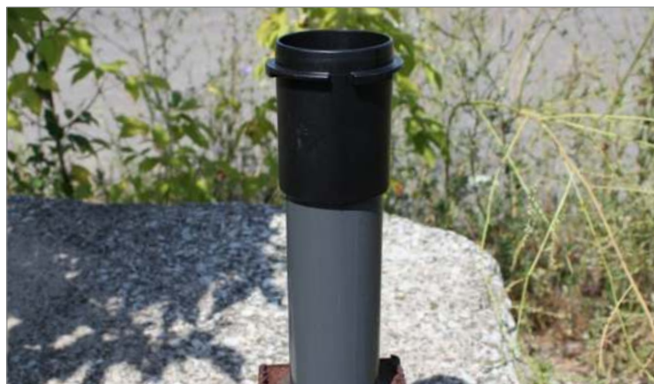
Install the well cap base on the well casing.
