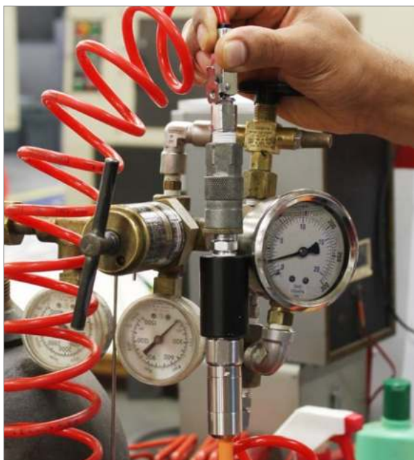
Figure 9-6 Nitrogen Gas Being Blown Through the Vented Cable
