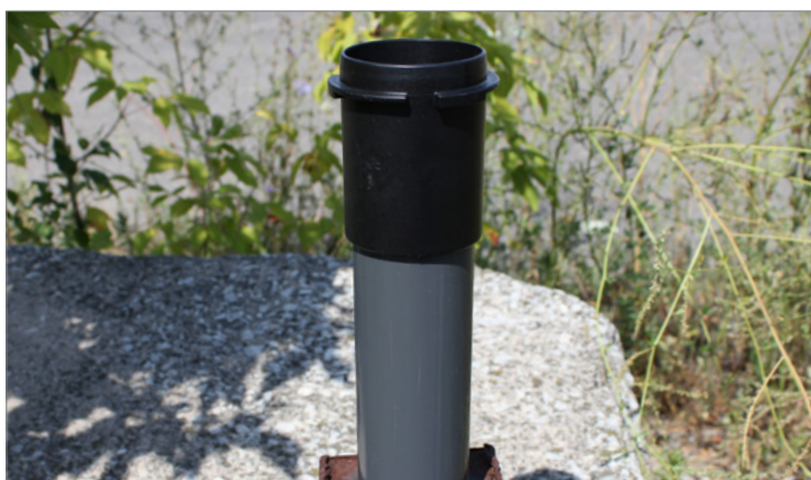
Install the well cap base on the well casing.
